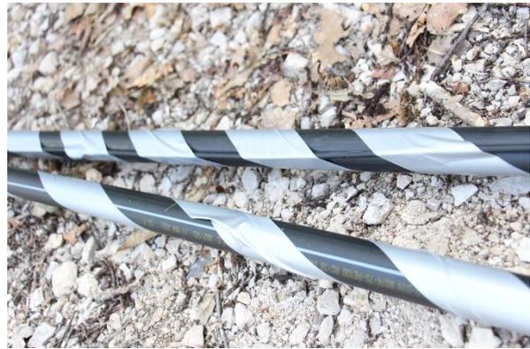
**Figure 2: Optical cable fixed on one U-tube of the double-U tube BHE**
