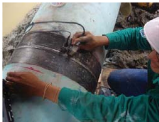
Figure 2. Welding pipe applied in section.
