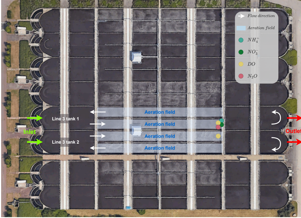
Figure 2: Aerial photograph of the 8 aeration tanks at the case plant. The sensor placement, aeration field and flow directions are indicated in tank 1 and tank 2 for line 3.
