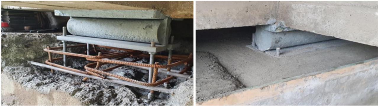
Figure 21. Cause, effect or both? Southeast roller bearing, before and after repair.
