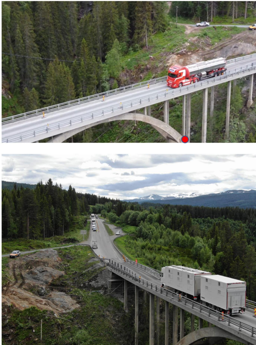
Figure 16. Repair done after April 2021, a ramp to offload the south abutment implied an elevation of a stretch of the road, picture showing northbound truck on top (location of sensor K marked by red circle), southbound on bottom. Photos: Kjetil Sletten.
