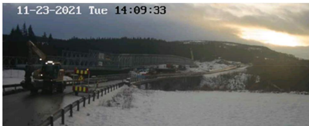
Figure 15. Two excavators crossing bridge cause an impulse on entry, giving rise to large horizontal responses in the first natural frequency, combined with high-frequency disturbance during crossing.
