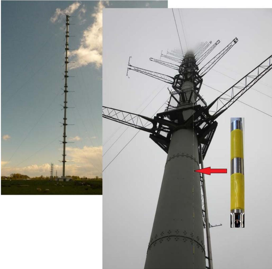
**Fig. 1.** View from the north of the entire KNMI-mast in Cabauw in summer, and, in the foreground, from the south and from below in autumn-fog with lower end of temperature T-sensor cable suspended along-side (the red arrow points at a T-sensor).
