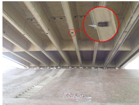
Fig. 3: Picture that highlights the placement of the sensors that are attached to the girders and bottom of the deck (from (Miao 2014)).
