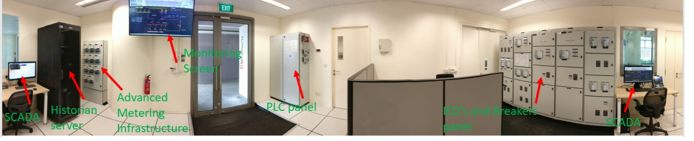
Figure 3: EPIC control room, 360-degree view. The picture shows different physical components including the SCADA workstation, IED and Breaker panel, PLC panel, Historian server, Advanced Metering Infrastructure (AMI) and the Monitoring screen.
