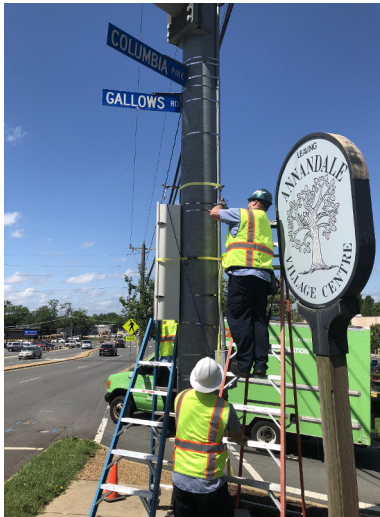
Figure 1: A typical NOVAArray sensor configuration. The detector is housed in the white box and mounted to a traffic signal post.
