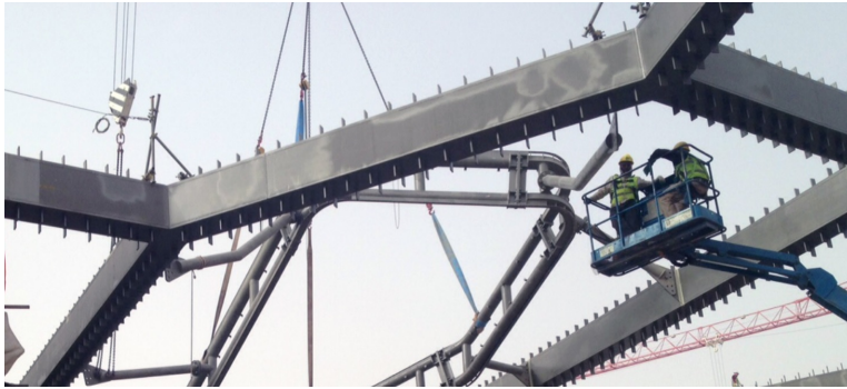
FIGURE 3. Connection of beams by rigid joints (source).
