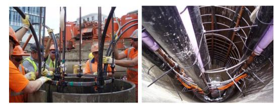
Figure 9: Installation of geothermal loop into the energy pile (courtesy of Kenichi Soga)
