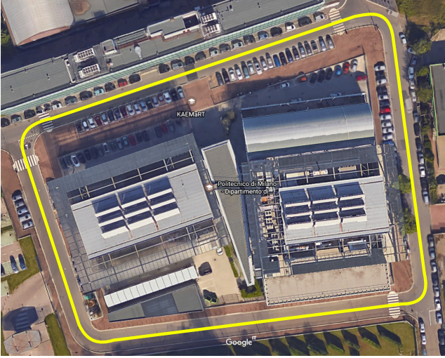
Fig. 10. Mechanical Engineering Department area
