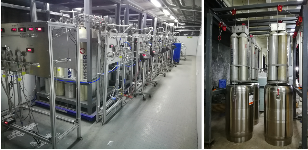
Figure 2. Xenon room temperature storage (Left) and LN2 emergency recovery system (Right) at CJPL-II.
