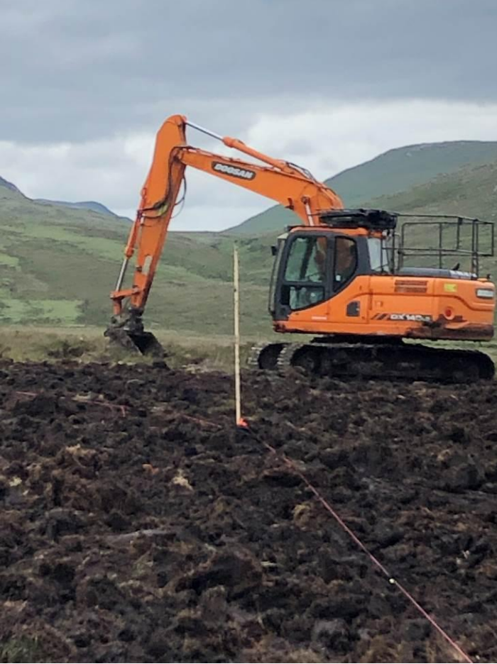
Figure A4. Wooden stake and three survey lines mark the center of the original impact crater for subsequent expeditions to extend the investigation into the granite bedrock below 6.5-m depth.
