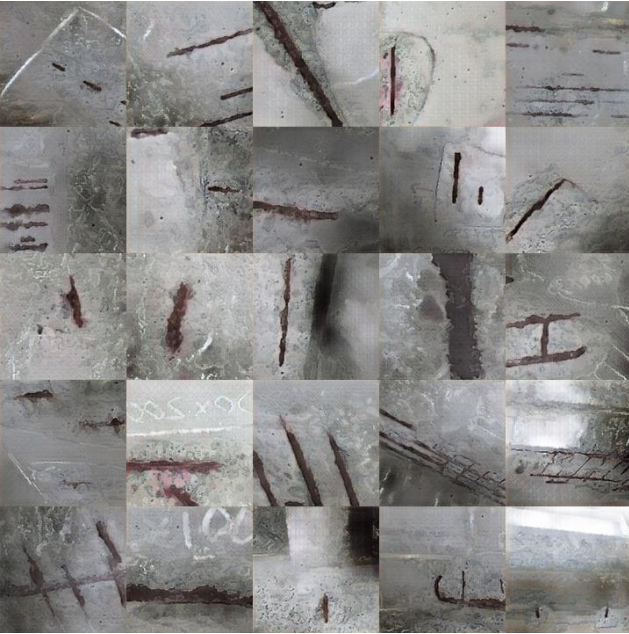
Figure 2: Generated images using synthetic augmentation using L1-Conditional GAN in case of rebar exposure at concrete bridge.
