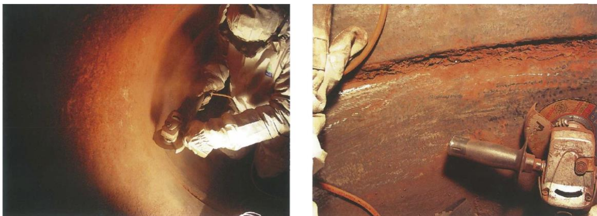
Figure 2: Operator inside a 1000mm diameter cast-iron pipe cleaning the pipe joint.
