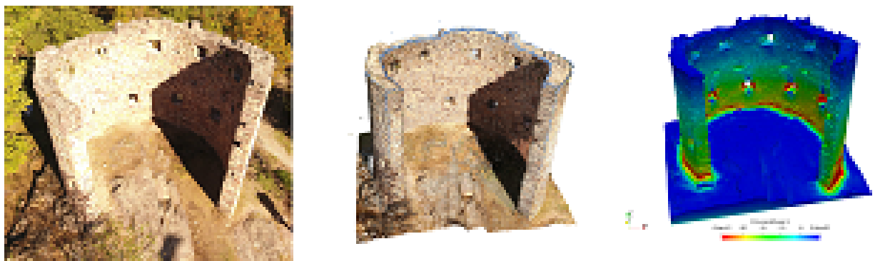
Figure 23: Tower ruin: photo taken by the UAV, point cloud and the maximum principal stresses computed by the FCM
