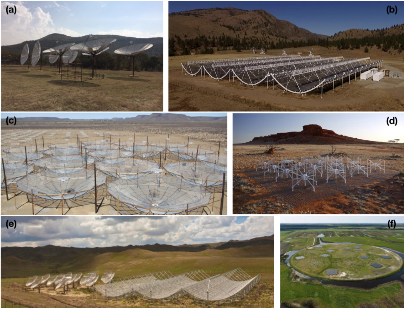
FIG. 24. A sample of relevant 21 cm interferometric experiments currently fielded: (a) 8-element HIRAX prototype array operating at 400–800 MHz [191]; (b) CHIME experiment operating at 400–800 MHz [213]; (c) HERA [214] operating at 50–250 MHz with PAPER [215] in the background; (d) MWA operating at 80–300 MHz [216]; (e) Tianlai [217] operating at 700–800 MHz; (f) LOFAR [218] operating at 10–230 MHz. EDGES [219] is not included because it is targeting a global signal. LEDA is relevant but not pictured [220].
