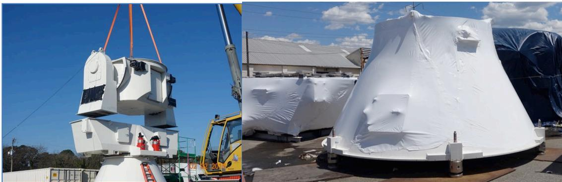
Figure 5: Left: Disassembly of the receiver cabin/yoke arms unit from the yoke traverse, before insulation work; Right: Shrink-wrap of the support cone with the azimuth bearing and lifting fixture integrated is in progress.
