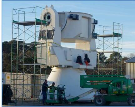
Figure 3: Elevation bearings installed, cabin mounted and aligned
