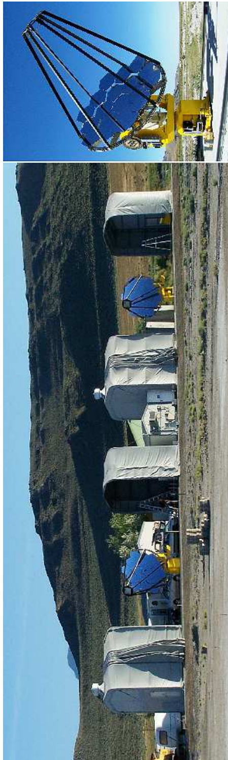
Figure 10: The StarBase 3 m telescopes are protected by buildings which can be rolled open for observation (left) The control room is located in a smaller building located between the two telescopes. Right: Close-up view of one telescope.
