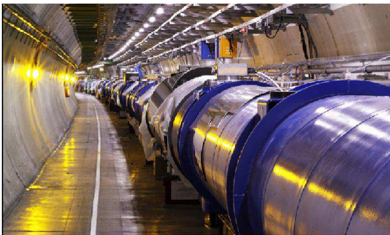
Figure 10. The LHC tunnel with its accelerating magnets.
