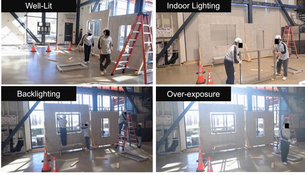
Figure 5. Illumination Variations. Sample lighting scenarios encountered during testing of Safe-Construct. The first row shows well-lit indoor rooms common in indoor construction; the second row presents backlighting and over-exposure, which reduces visibility and presents a darker appearance.
