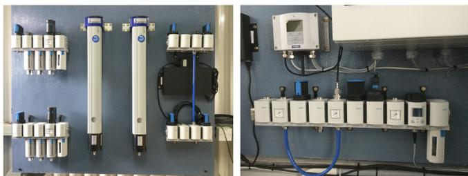
**Fig. 6.** Double air filtration systems located in the compressor room (left). A separate equipment combines air from each system, providing further filtration, pressure regulation and sensors (right). The latter equipment is located in the telescope control room.
