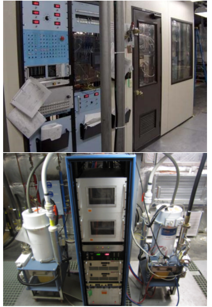
FIG. 36. The 20 kV High Voltage enclosure and controls above and a pair of 10 kW IOTs with their controls below.
