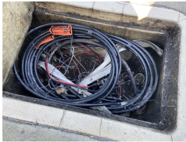
Fig. 3. An example photo showing fiber spooling.
