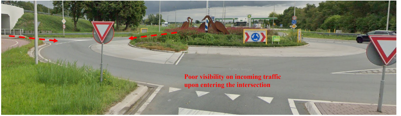
Fig. 6. The visibility condition when entering the first roundabout on the test route. Vehicles entering from two other directions, represented by the arrows, only become visible at a distance of approximately 30 m. Image source: Google Street View
