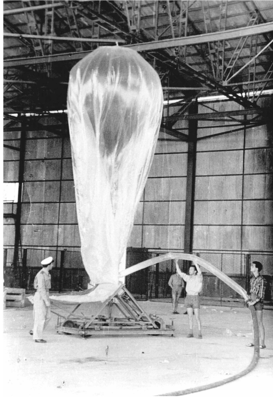
Fig. 5 The stratospheric balloon, with a volume of about 9 000 cubic meters, launched from the Cagliari Elmas Airport (Sardinia, Italy) in the early 1950s. Courtesy of P. Ubertini.
