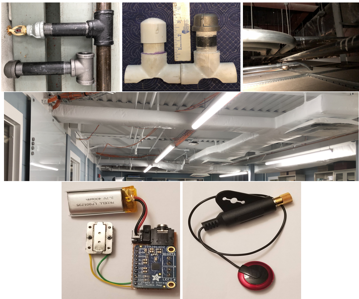
Figure 1: Pipes, Fittings, and Hardware. (top left) In spite of the wide variety of colors, textures, and sheens, all of these are black steel except the sprinkler head itself, the bright silver galvanized steel bell fitting attached to the sprinkler head, and the faux T fitting at upper right. (top center) Pipe length required to hold receiver, mocked up in 1 inch diameter PVC and black steel. (top right) Typical mechanical systems above a suspended ceiling in new construction. (middle) Typical mechanicals below a finished ceiling in old construction. (bottom left) Best transmitter tested (Adafruit transducer and amplifier). (bottom right) Best receiver tested (Traderplus).
