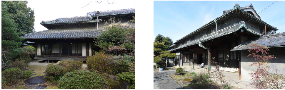
Figure 7: Exterior photos of house with pantile roofs.
