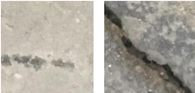
(a) An image without any cracks in it, labelled "Negative" (b) An image with a crack in it, labelled "Positive"
