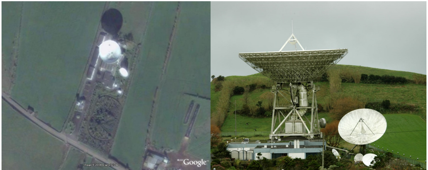
Fig. 2. SATCOM Earth Station in São Miguel (Azores) – Intelsat Standard A 32-metre parabolic antenna, Altice Portugal. We can see the waveguide system below the dish.
