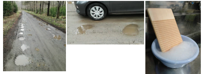
FIG. 1. Left: Road corrugation on unpaved road. Terrain undulations are clearly identified due to the rainwater collected in the depressions. Middle: Comparison of the period of corrugation with vehicle dimensions. Right: Photograph of a washboard.
