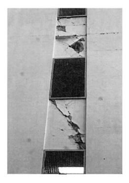
Figure 32. Failure of spandrel beams in Northridge earthquake [23]
