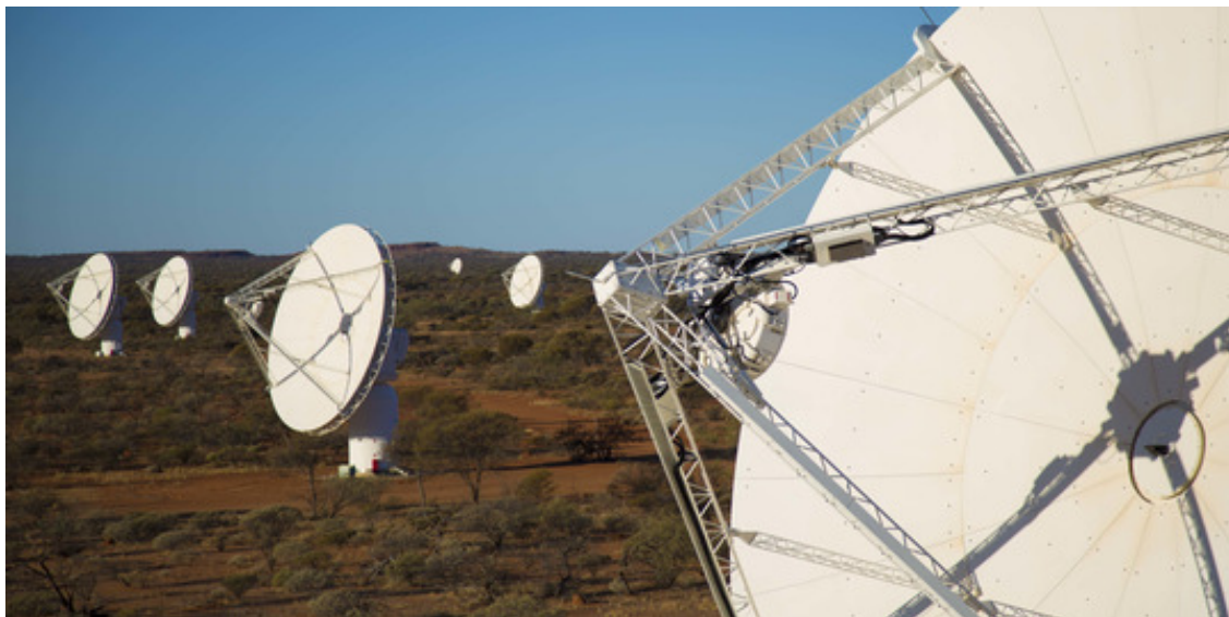
Fig. 4 ASKAP antennas equipped with MkII Phased Array Feeds, 2017. — Photo credit: CSIRO.
