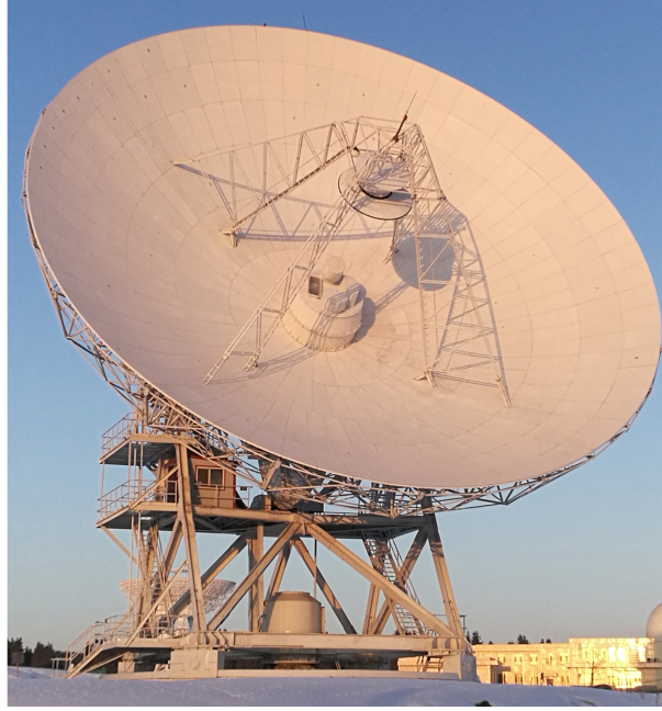
Fig. 6: The image of a 25 m shaped Cassegrain antenna.
