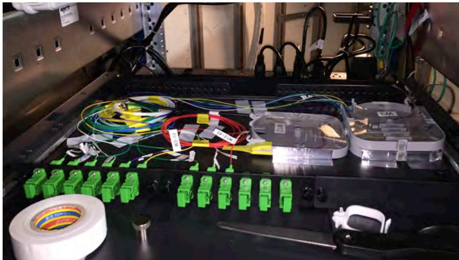
Figure 36. Fiber termination chassis located in terminal racks. This photo is of the receiver cabin left rack, which provides terminations for cables W2, W3, and W12.
