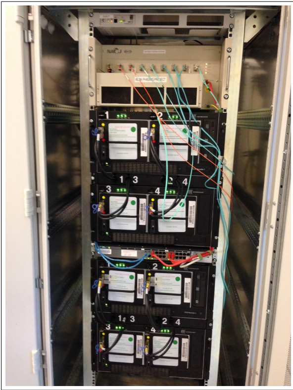
FIG. 8.— Recorders 1 and 4 installed in the designated ALMA OSF computer room rack. The OFLS unit is mounted at the top. Between the recorders is the network switch which connects the recorders to the AOS network and also provides a private network between the recorders.
