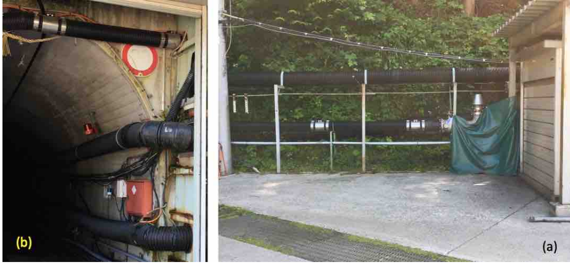
Figure 3.5: Air lines for KamLAND (lower) and SuperK (upper), (a) near pump buildings, and (b) entering mine access road.
