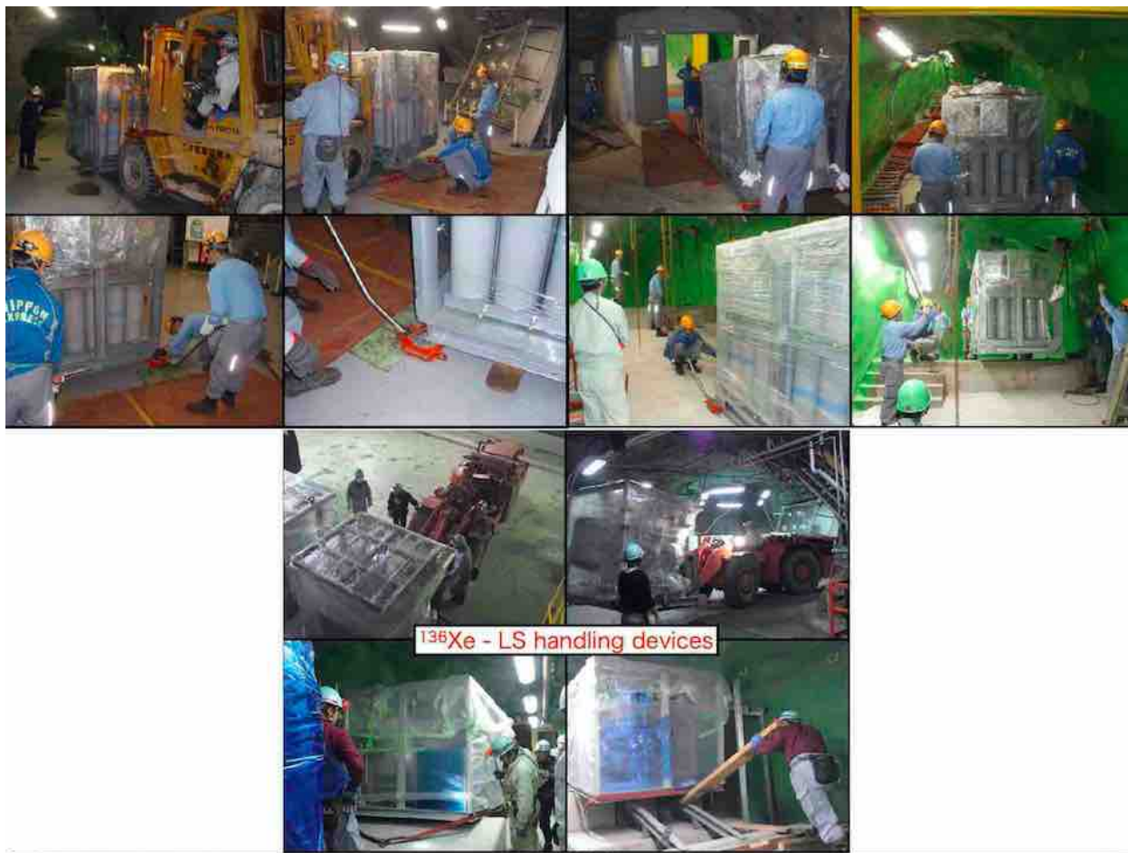
Figure 2.13: Photos from installation of the xenon systems for the Zen experiment. Note the diversity of rigging equipment employed, from forklifts to hydraulic lifters. In particular, note the use of ceiling hooks (second row right side).
