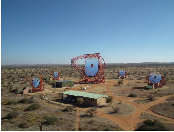
Figure 1 – Left: Photograph of the H.E.S.S. gamma-ray observatory in its final configuration of four 12 m telescopes combined with a central 28 m telescope. Right: Schematic view of the H.E.S.S. alert reception system allowing to receive alerts from observatories covering all wavelengths and astrophysical messengers. From 3 .
