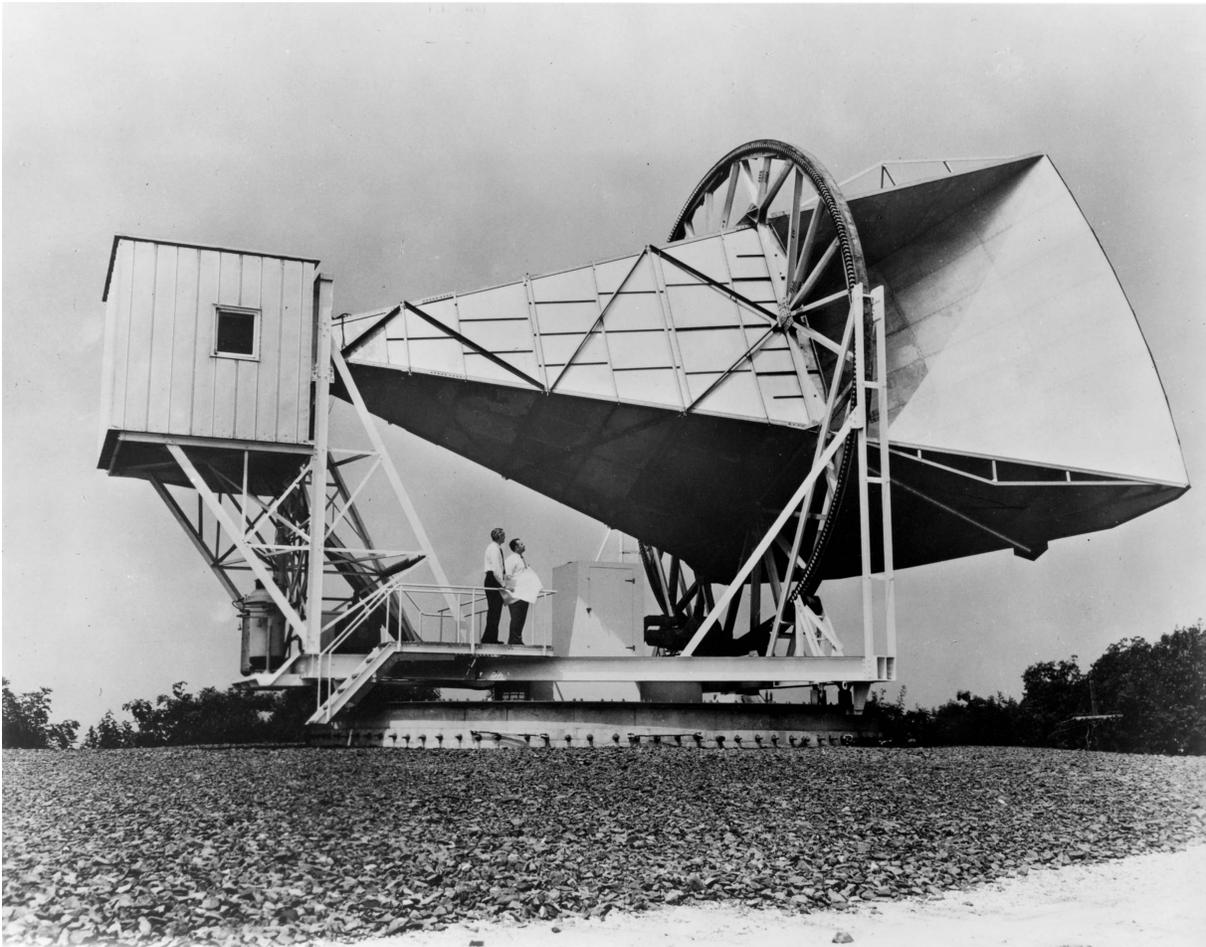
Figure 1: **Horn antenna used in 1964 by Penzias and Wilson to discover the CMB.**
