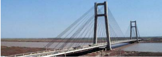
Figure 8 Photo of the Tianjin Yonghe Bridge
