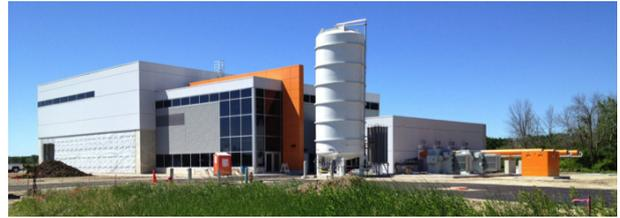
Figure 3: The new MC-1 building at Fermilab, where the muon g-2 storage ring is being reassembled in the larger part to the left. The part to the right houses the counting room, electronics, etc., with cryogenics services further right. (Image credit: Fermilab.)
