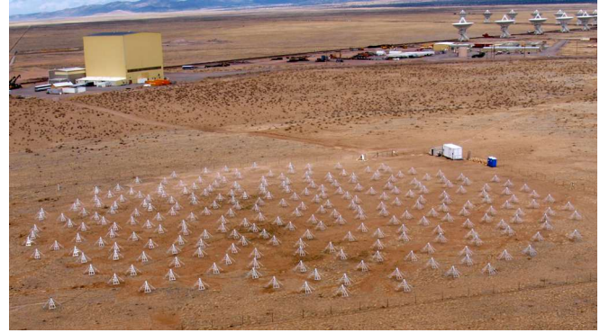
Fig. 1. LWA1. The white cargo container beyond the station array is the electronics shelter. Visible in the background is the center of the VLA.
