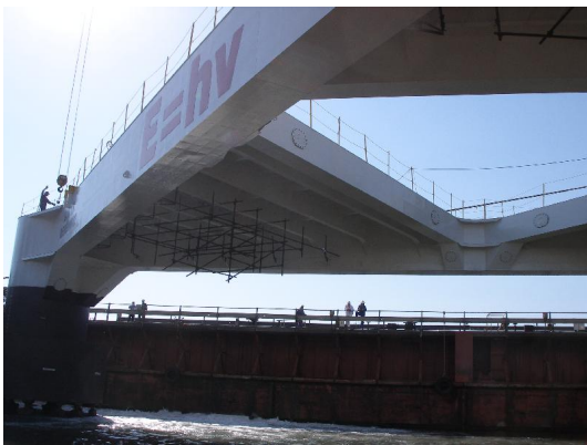
Figure 24. Photograph of the Delta Berenike platform in the final phase of its construction.
