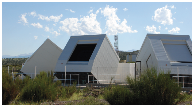
Figure 3: Photo of the three HEAT buildings in tilted mode.
