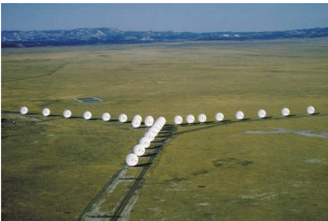
FIG. 1.— An aerial photograph of the VLA in its most compact “D” configuration, with maximum baseline 1.0 km. The array can be reconfigured by moving the antennas to more distant pads via the rail lines visible in the photograph.
