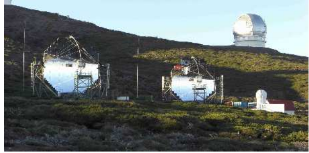
Fig. 1: The two MAGIC telescopes in April 2009. The first telescope, on the left, operates regularly since 2004. The second telescope can be seen on the right. The frame, mirrors, active mirror control and drive hardware were installed in Summer 2008.
