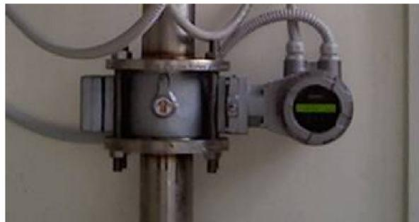
**Fig. 1: Electromagnetic flow meter. Accuracy  $1 \times 10^{-5} \text{ m}^3/\text{s}$**
