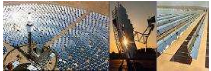
Figure 8: Concentrated solar systems. For the system in the middle photo the efficiency for producing ac electricity is ~30%.
